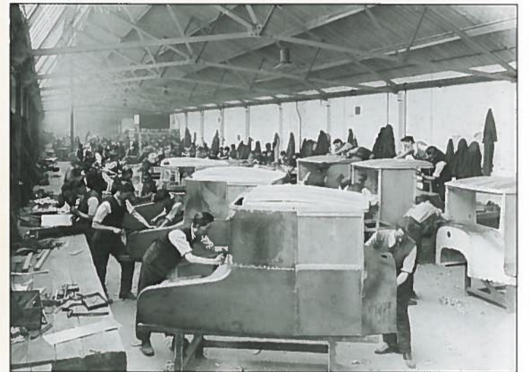
Workers finish off wooden body frames for the panelling. In the sheet metal department, the wooden bodies were panelled with metal sheets (1925).
